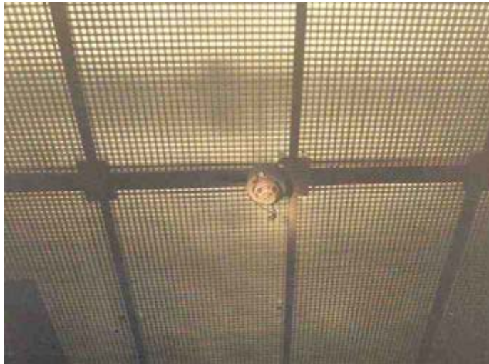
Figure A.4: Example of a Grated Ceiling Found in Main Control Room
