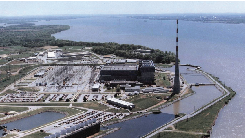
Aerial view of Browns Ferry Nuclear Plant (TVA File photo)
