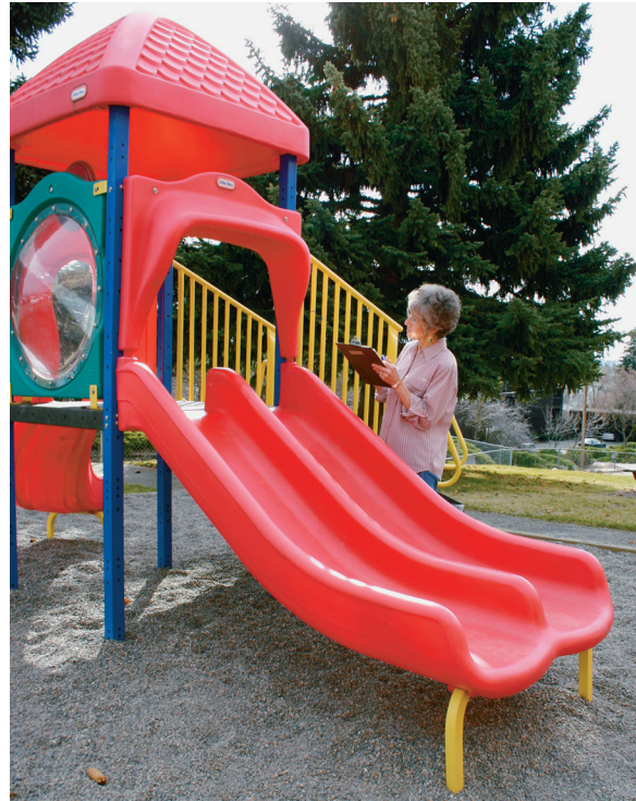
● Figure 10-4 Assess the childcare center's environment for safety hazards. Check the area around playground equipment, making sure there are wood chips or cushioned tiles under the equipment. Inspect the playground equipment for protruding screws, loose nuts and bolts, and instability at least monthly.
