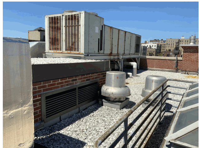
Roof 1 - Northwest View
