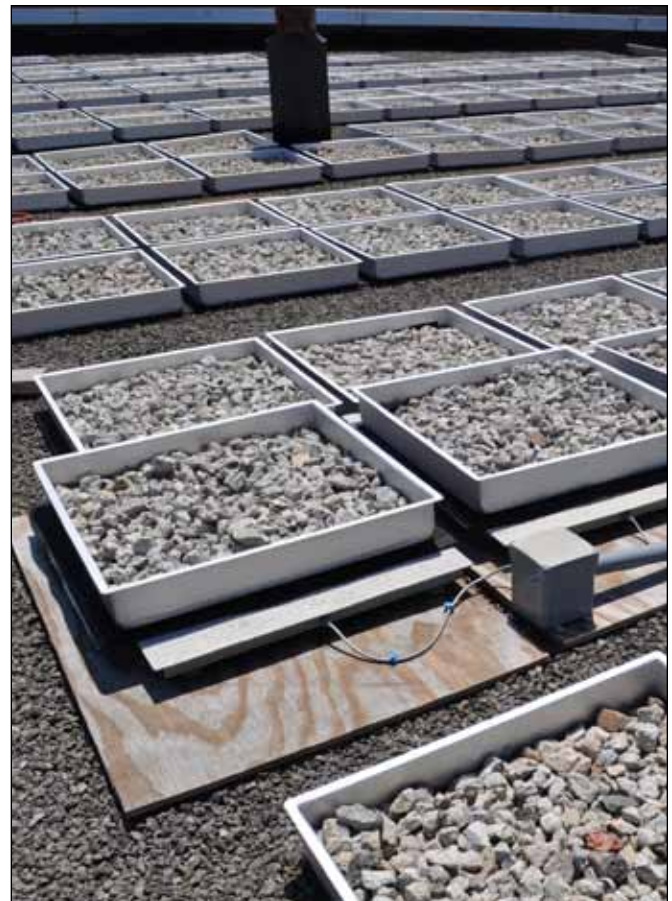
DEP installed weight scales in three trays to determine evaporation rates, drawdown times, and average and peak flow rates.
