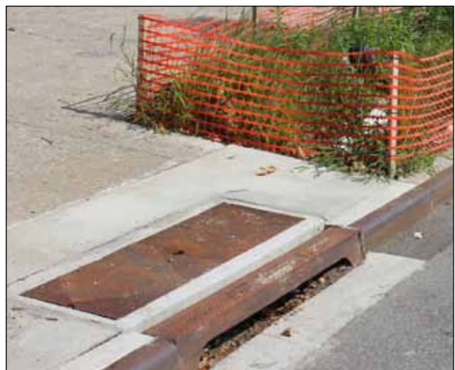
At the Eastern Parkway ETP, DEP moved the inlet catch basin three feet upstream.
