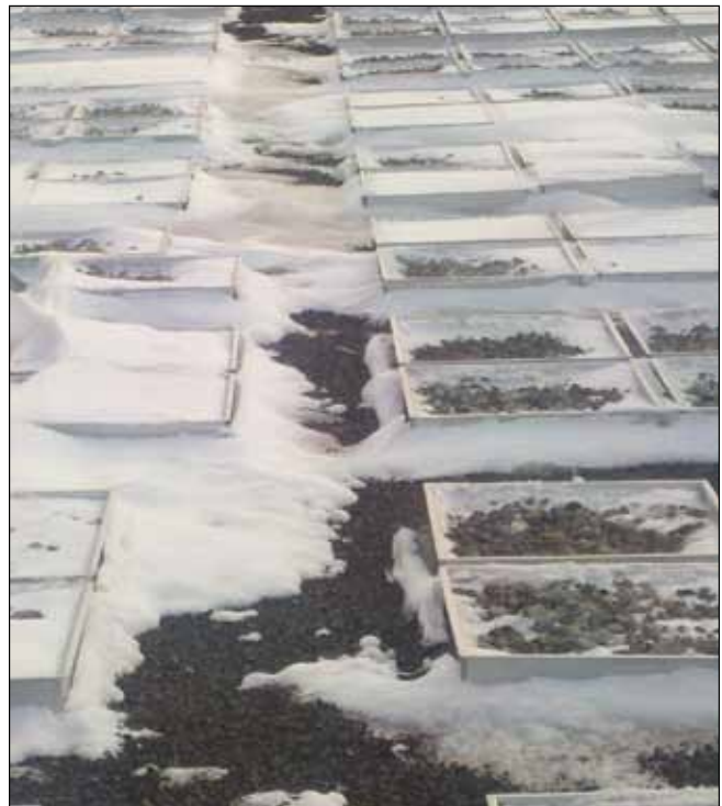
Future research at this site will measure the performance of the different blue roof technologies year round.
