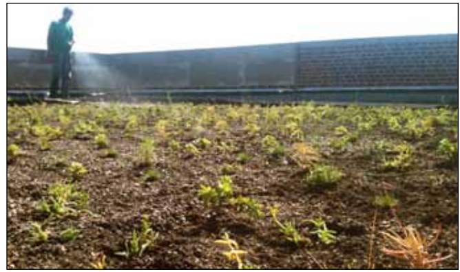
Green roofs have higher maintenance costs because they require weeding, replanting, and irrigation.
