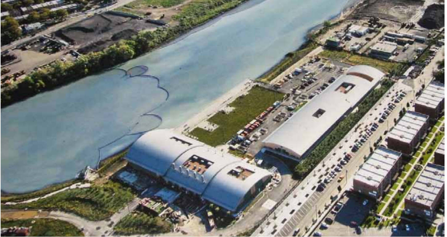
The Paerdegat Basin CSO Detention Facility, a cost effective grey infrastructure investment, can store up to 30 million gallons of untreated wastewater at a time.
