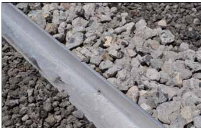
In the third quadrant, DEP installed check dams that restrict the flow of stormwater to the drain by forcing the water to flow through small orifices drilled into each dam.
