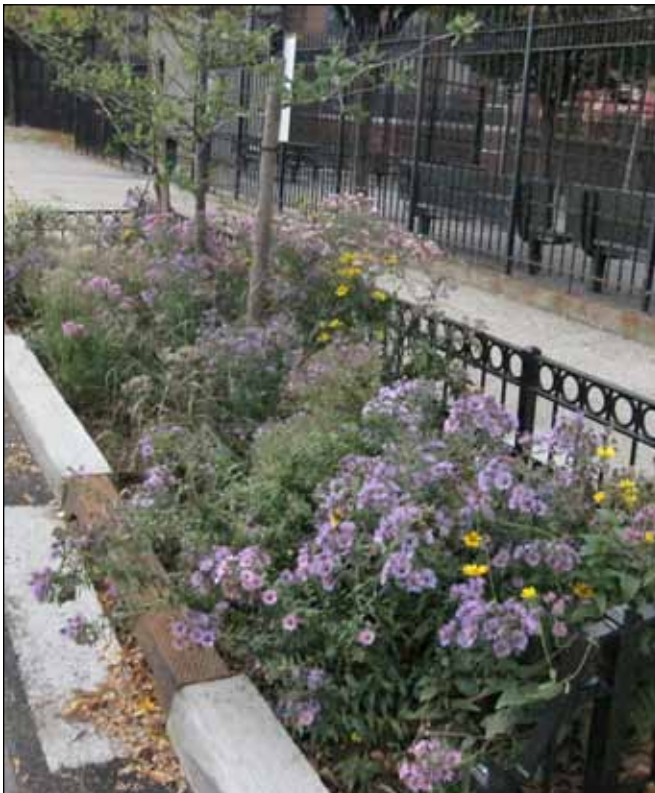
ETPs are 20 feet long, five feet wide, and 4.5 feet deep. ETPs have two subsurface layers: the top layer is made up of two feet of engineered soil, while the bottom layer contains 2.5 feet of gravel, recycled glass or storage chambers.
