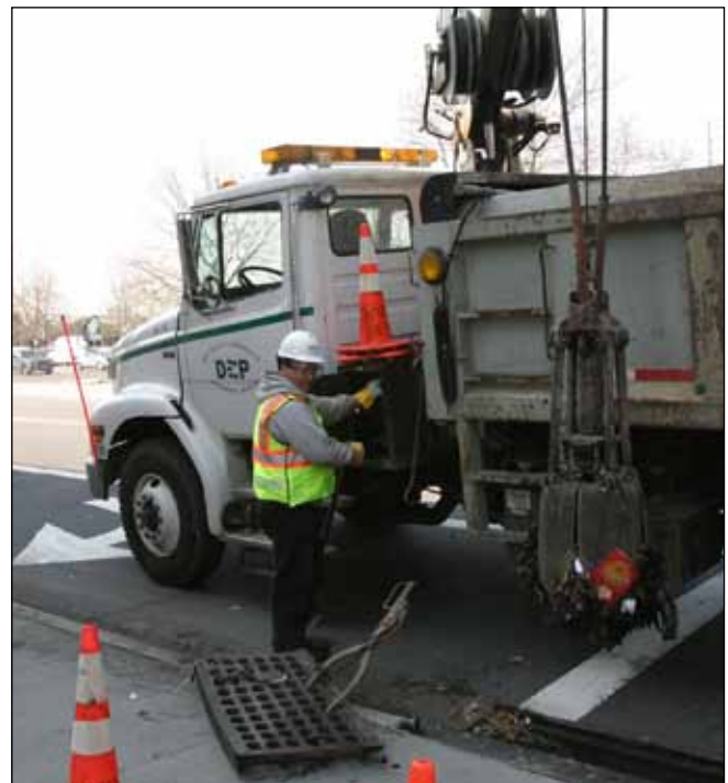
Cleaning catch basins increases the capacity of the sewer system.
