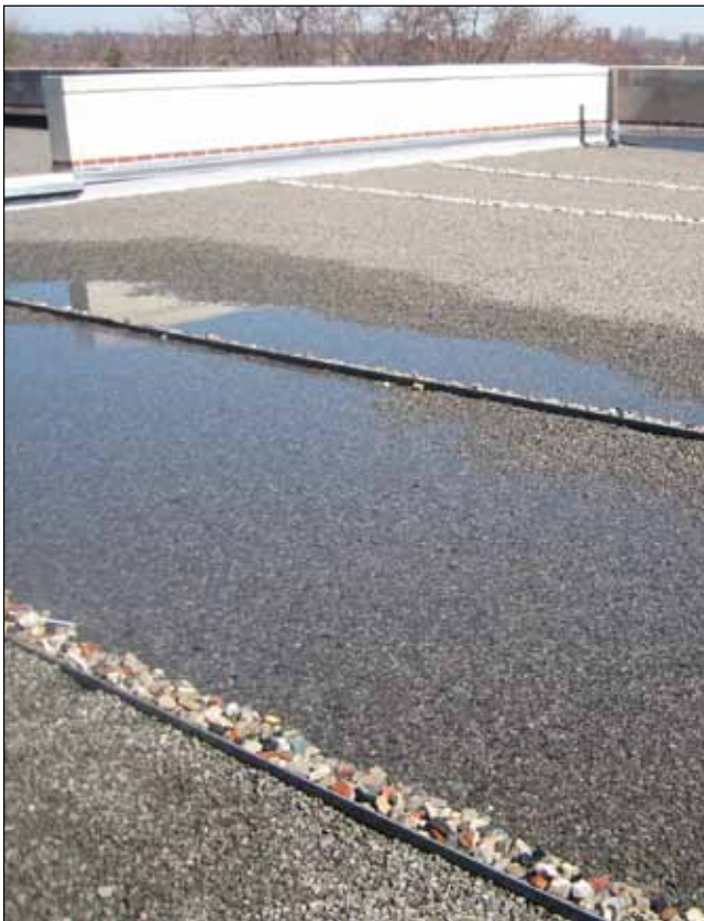
By building a blue roof and a green roof on the same building, DEP can determine which technology is most effective at managing stormwater.
