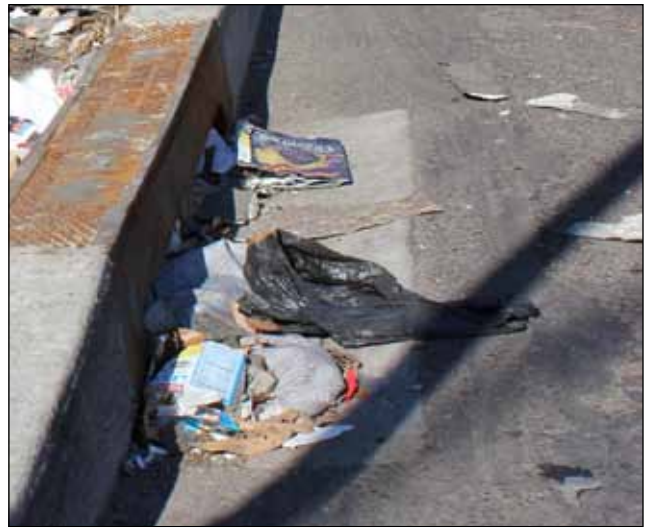
Litter often clogged the original inlet design, causing stormwater to bypass the ETP or SSIS completely.
