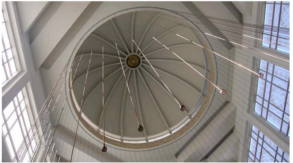
Looking up to the dome above.
