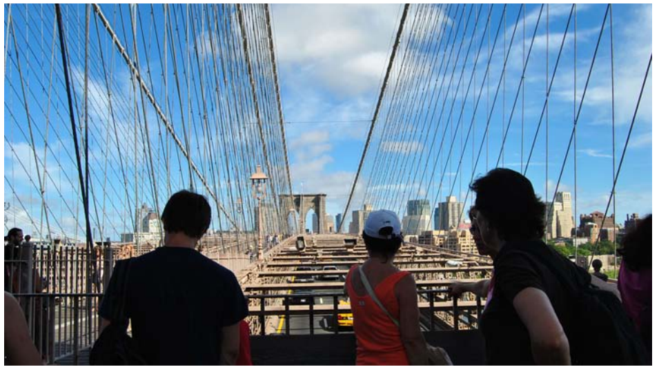
View from the middle of the bridge.
