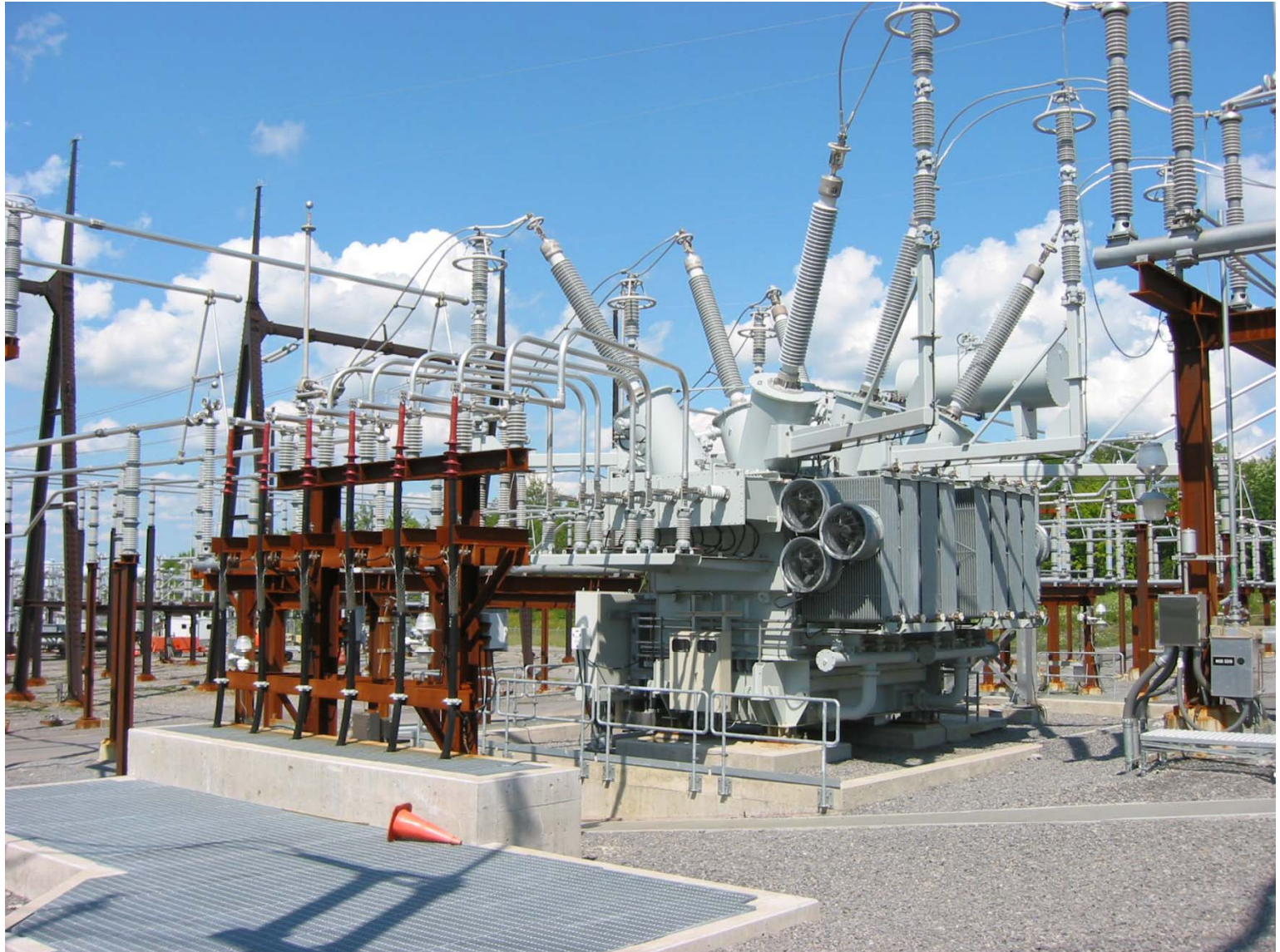
Future Renewable Electric Energy Delivery and Management Systems Center
