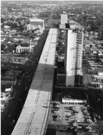
I-45 and Pierce elevated, Photo courtesy TxDOT Library
