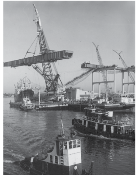
Construction on Houston ship channel bridge, Photo courtesy TxDOT Library
