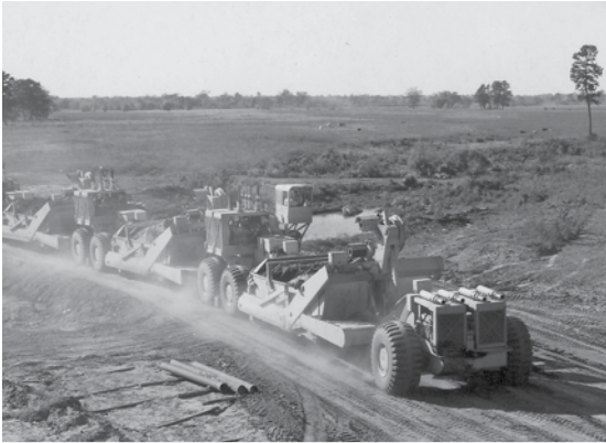
Earth moving machines in District 10 on I-20, Photo courtesy TxDOT Library
