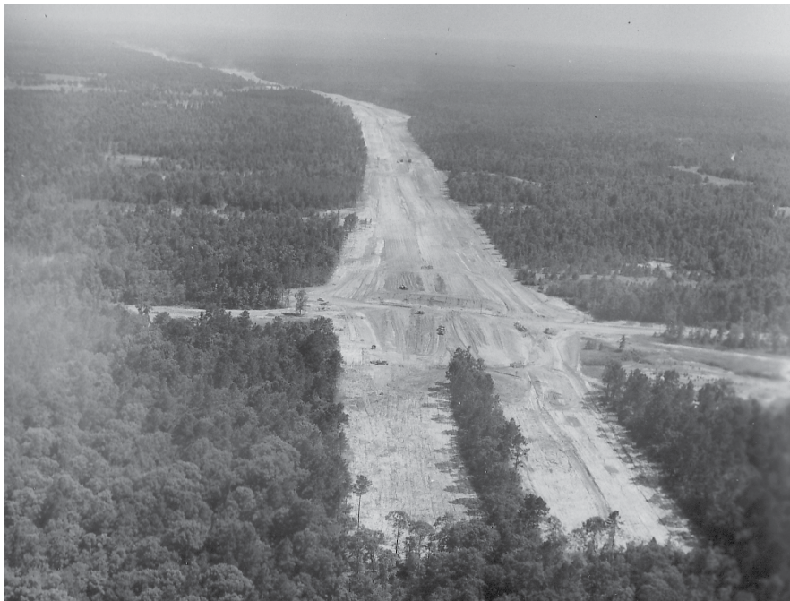
I-45 North of Conroe under construction, Photo courtesy TxDOT Library
