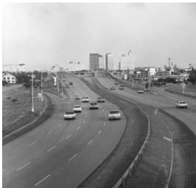
I-37 leading into Corpus Christi, Photo courtesy TxDOT Library
