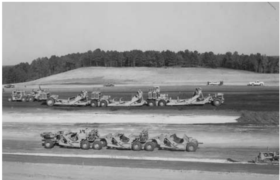
Earth moving machines on I-20, Photo courtesy TxDOT Library
