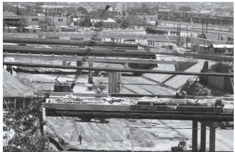
Construction in El Paso, Texas, Photo courtesy TxDOT Library
