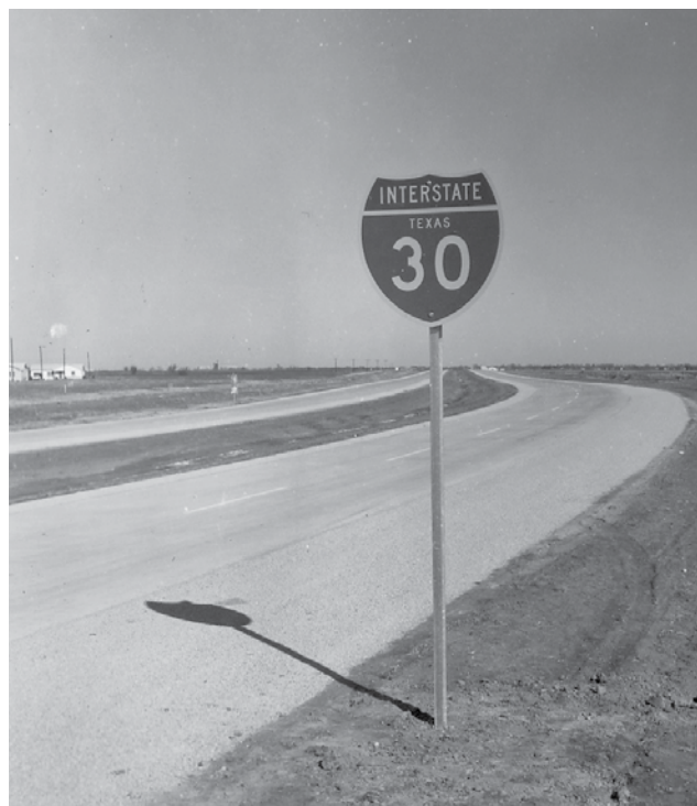
I-30, Greenville; first interstate sign erected, Photo courtesy TxDOT Library
