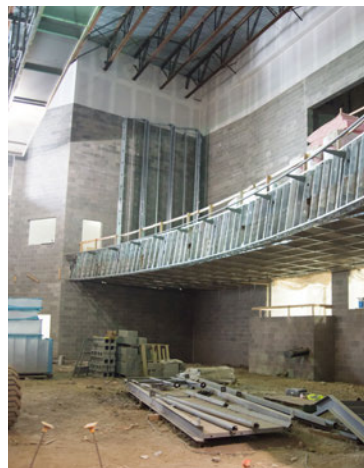
Balcony of 800 seat auditorium
