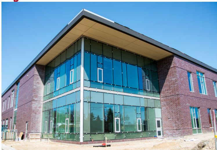
Exterior windows and brick
