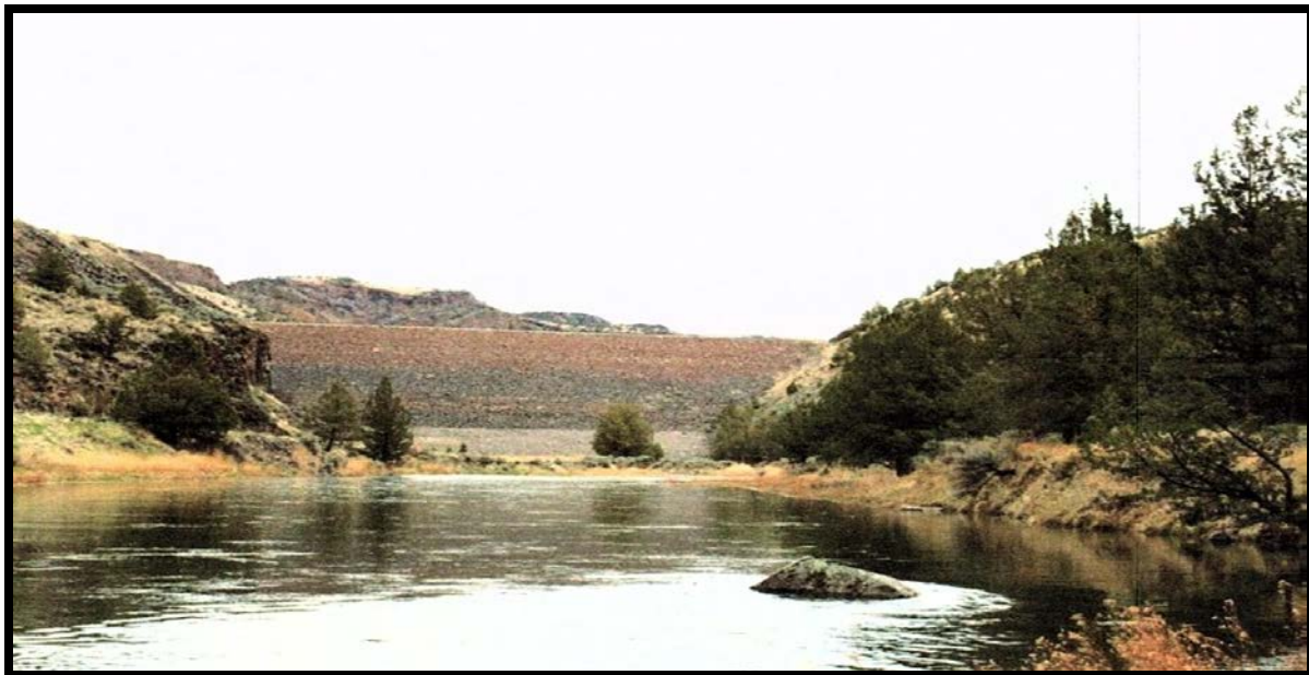
Figure 1. Downstream View looking upriver to Bowman Dam. (Source: PGE 2013)
