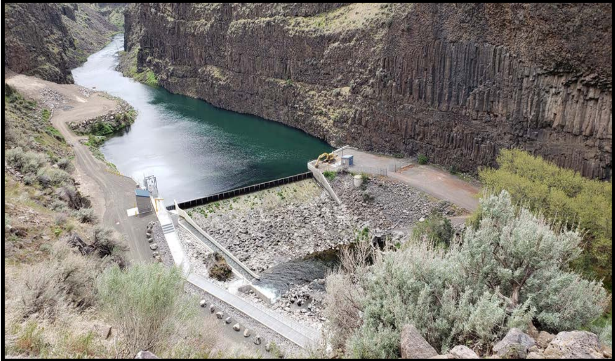
Figure 13. Opal Springs Dam Fish Ladder Recently Completed (November 2019) Passage Facility (Source T. Porter ODFW)
