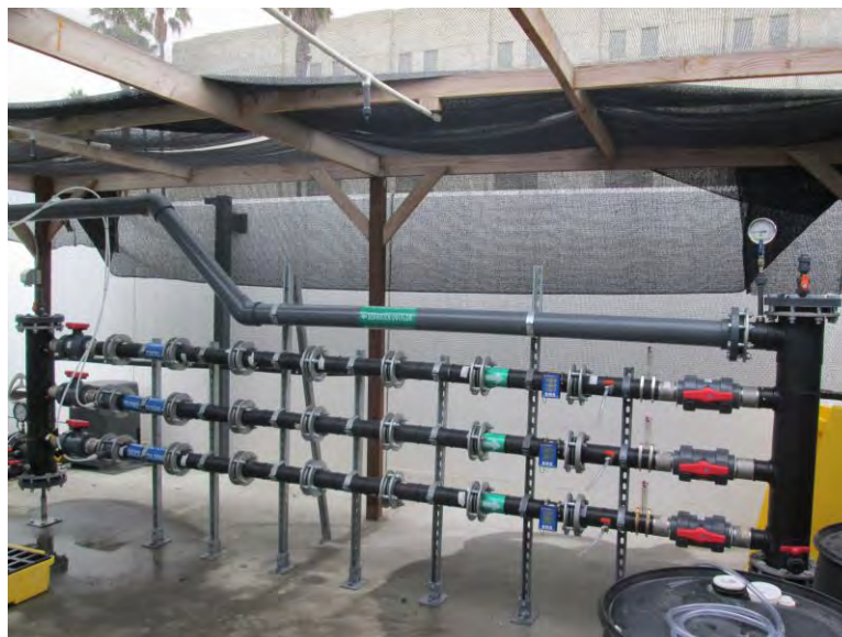
Close-up of the Pipe Test Runs
