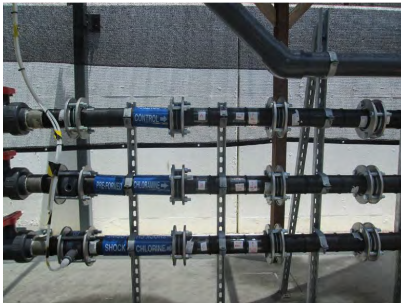
Close-up of Individual Pipe Spools
