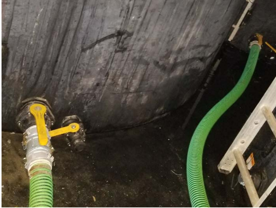
Photo 1 – 2x Leachate Tank Interconnecting Pipe Installed.
