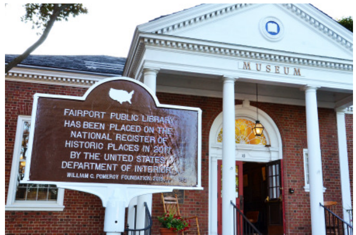
Provided through a grant of the William C. Pomeroy Foundation, the beautiful new historic marker is a welcome addition to the grounds of the Fairport Historical Museum.
