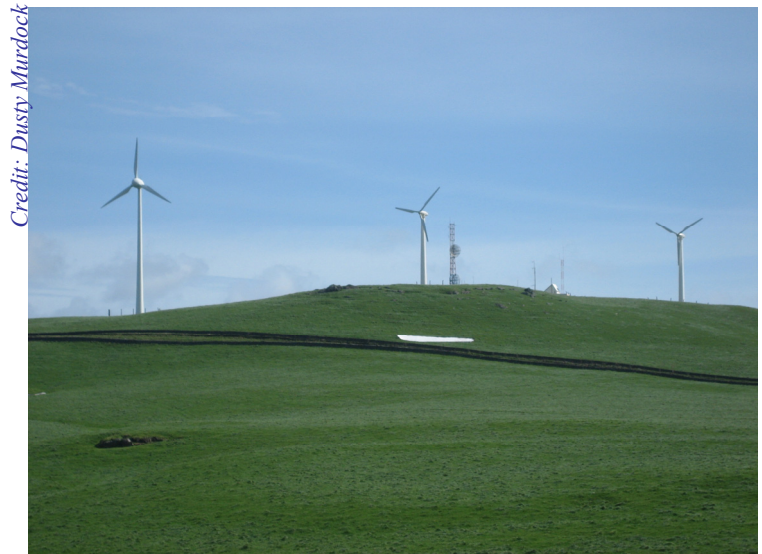
A wind development engineer spends some time in an office, using a computer to design and build power electronics that connect a wind turbine to a power grid. Most of his/her time is spent out in the field, in remote locations such as this island off the coast of Portugal.
