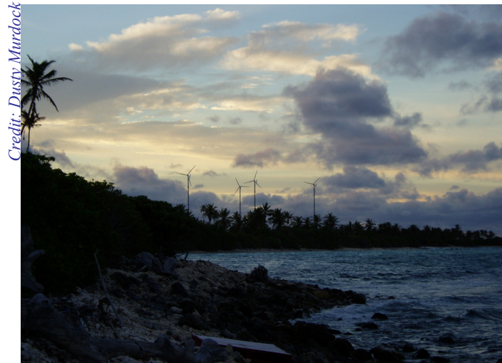
Dusty spent several weeks living on one of the remote Cocos Islands, while interfacing these four wind turbines to the power grid.
