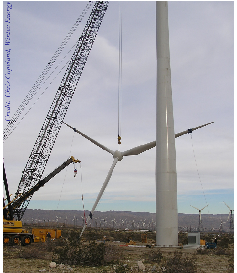
A key person on the wind farm construction team, a crane operator lifts the blades onto a wind turbine.
