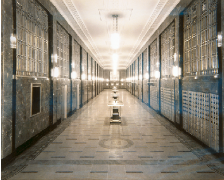
Lobby of the Nashville Post Office. Photograph. Marr & Holman Collection, Tennessee Historical Society, Tennessee State Library & Archives
