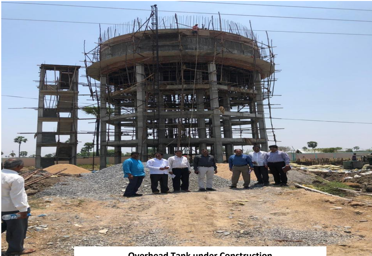
Overhead Tank under Construction
