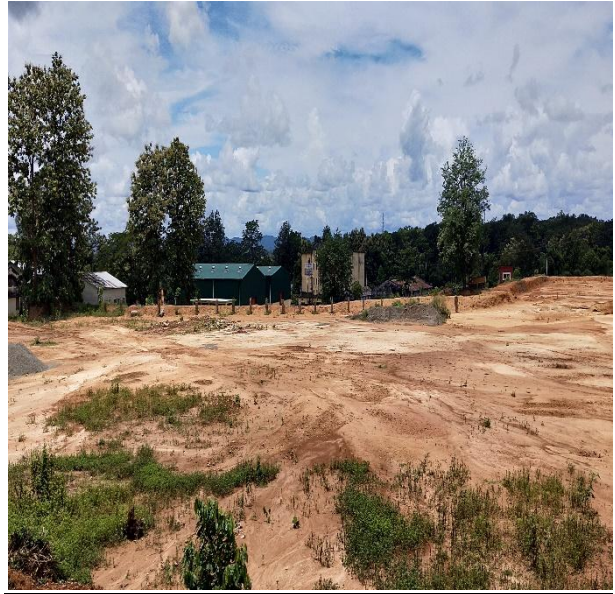
Leveling of sloping land
