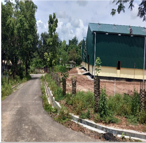
Constructed road, drainage & greenery
