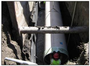
There were restraints on the design slope of the sewer and therefore field control of grade was critical.
