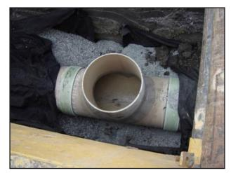
The design used HOBAS Tbase manholes with pressure tight lids.
