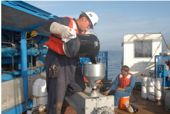
Figure A.7: Splice box being filled with No-Void
