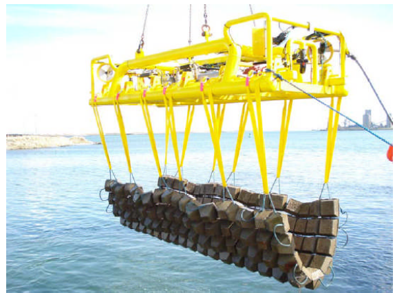
Figure 5.7: ROV deployment of concrete protection
