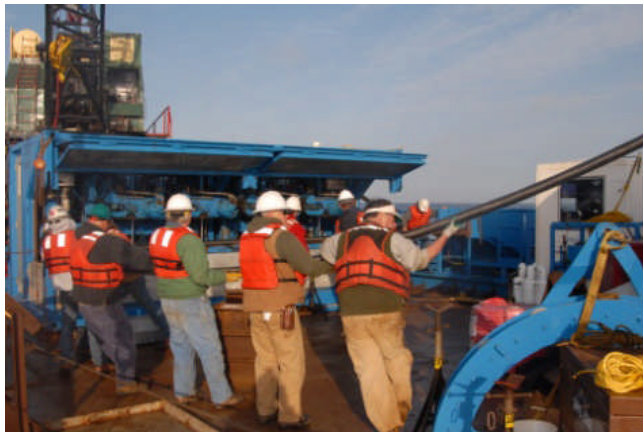
Figure A.9: Pulling cable
