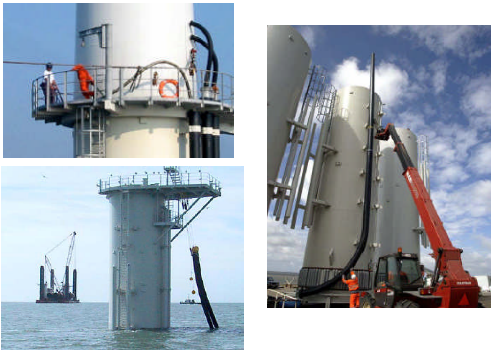
Figure 9.13: Photos of the Installation process (Source: Elsam 2002)
