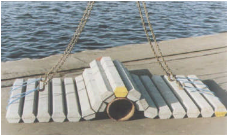
Figure 5.8: Concrete mattress in place protecting pipeline from cable laid above it.
