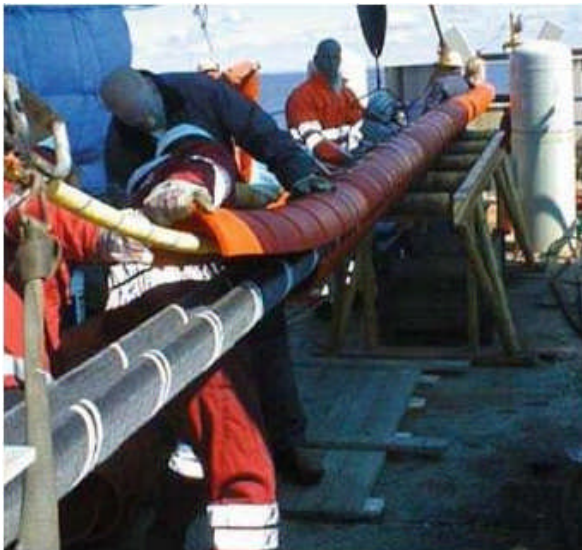
Figure D.11: Protective Plastic shells
