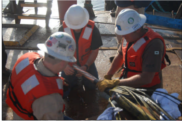
Figure A.6: j Splicing with the expert Jointers
