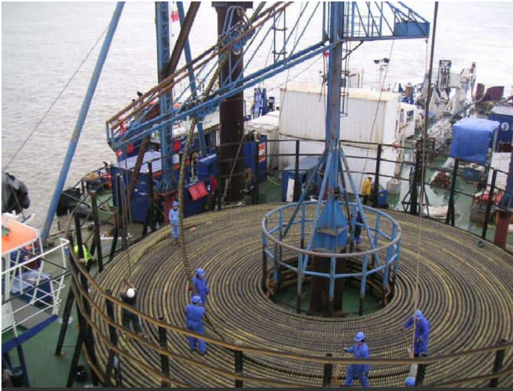
Figure D.10: Coiling Submarine Cable prior to Deployment
