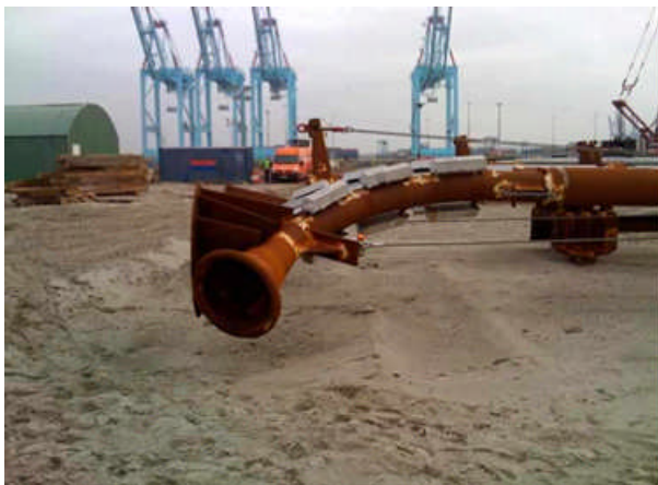
Figure 9.12: J-tube laid on side during construction
