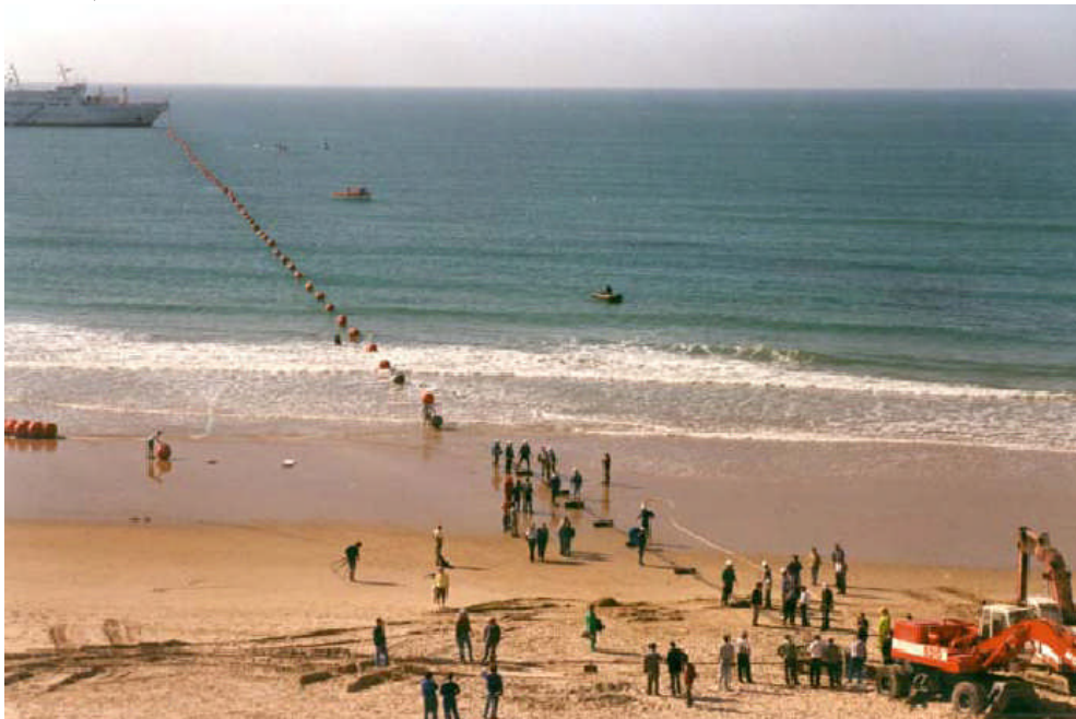
Figure 9.15: Buoyed Line with cable being brought ashore.
