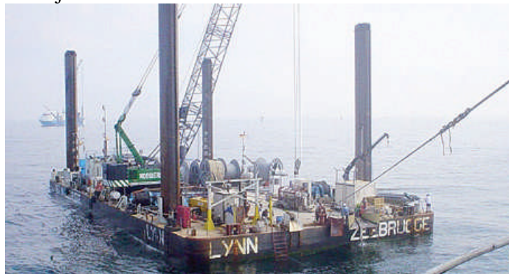
Figure 9.1: Cable laying within a wind farm (Courtesy Nexans)
