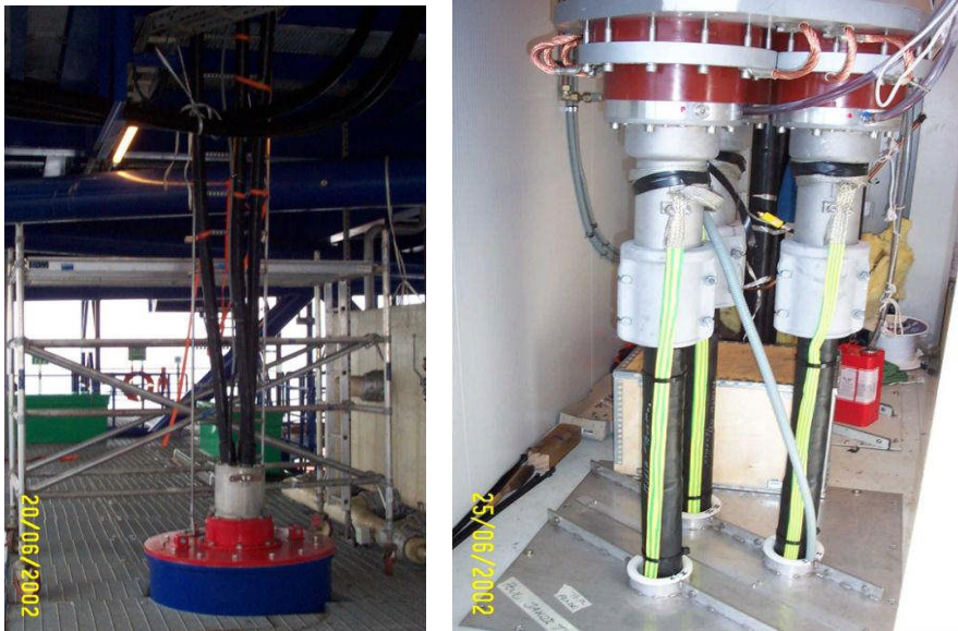
Figure 4.5: Cable Terminations at Horns Rev 2 (Courtesy Nexans)
