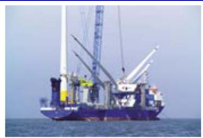
Construction of Kentish Flats @ Elsam
