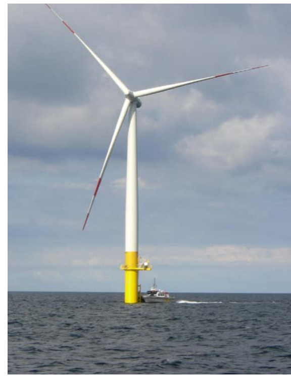
Baltic-1 2.3-MW Siemens fixed-bottom wind turbine in Germany; 2010 monopile substructure. Photo by Walt Musial
