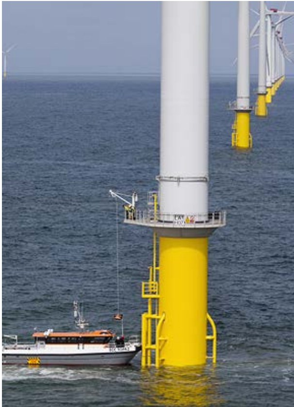
Photo by Siemens, NREL 277866
