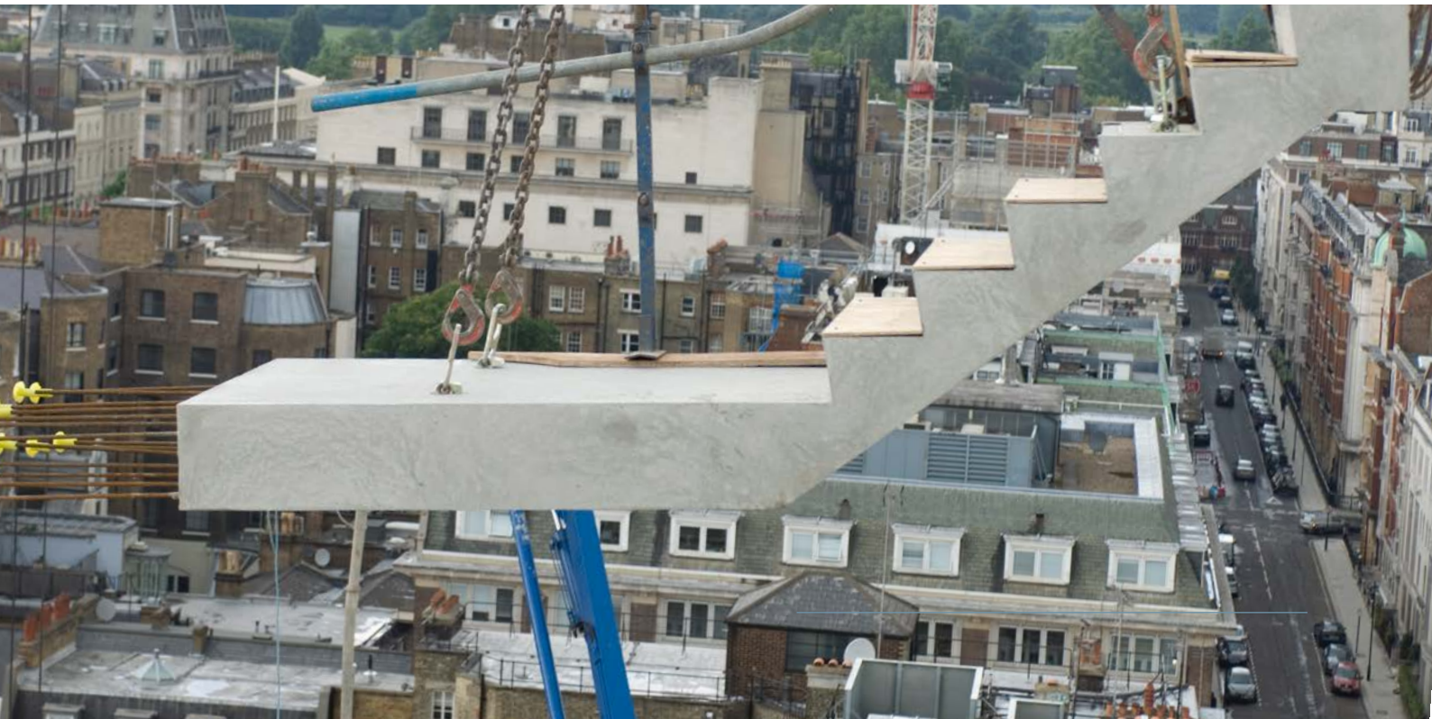
Precast concrete stairs at BBC HQ Building, London. Photographer: Grant Smith.
