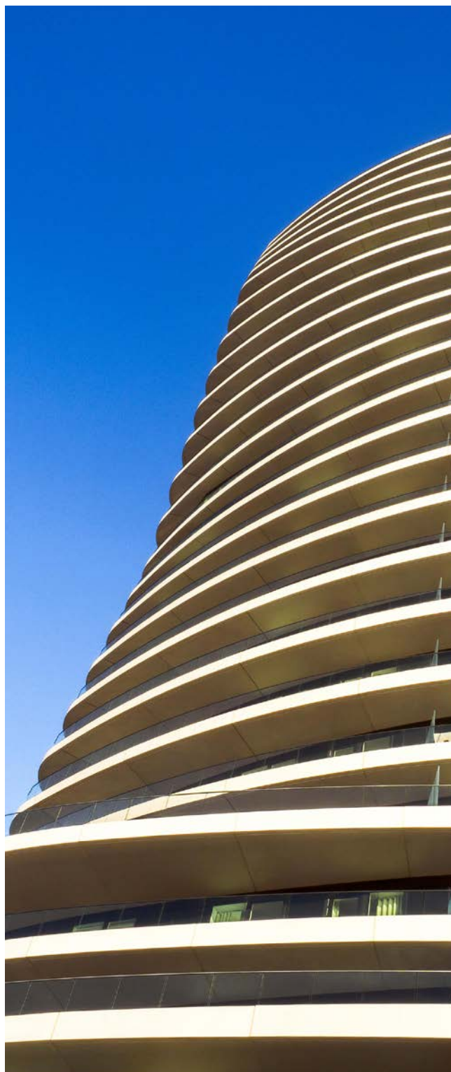
Lombard Wharf, Battersea features precast concrete wrap-around balconies which provided an elegant and robust solution © Alamy.
