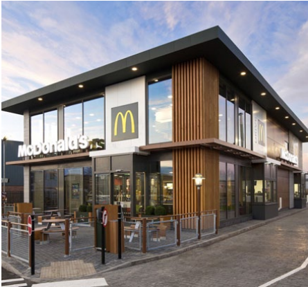
Fig 3.7 - An offsite McDonald's restaurant by Elliot Group
