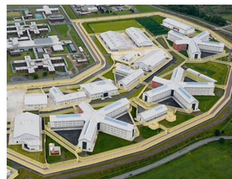
Fig 4.1 - HMP Oakwood: 76,000 man hours of construction activity saved from using pre-cast solutions. Capital savings estimated at £5m.
