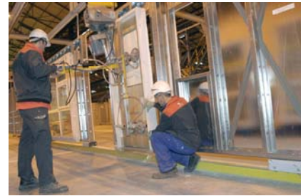
Steel frame and door set being erected
