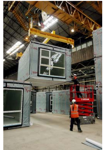
Finished module being stacked ready for delivery to site
