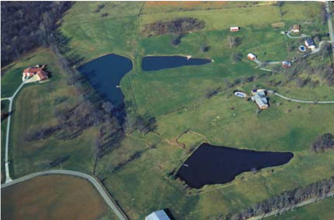
Aerial view of excavated ponds
