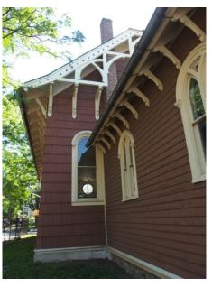
Detail of Brackets and Truss
