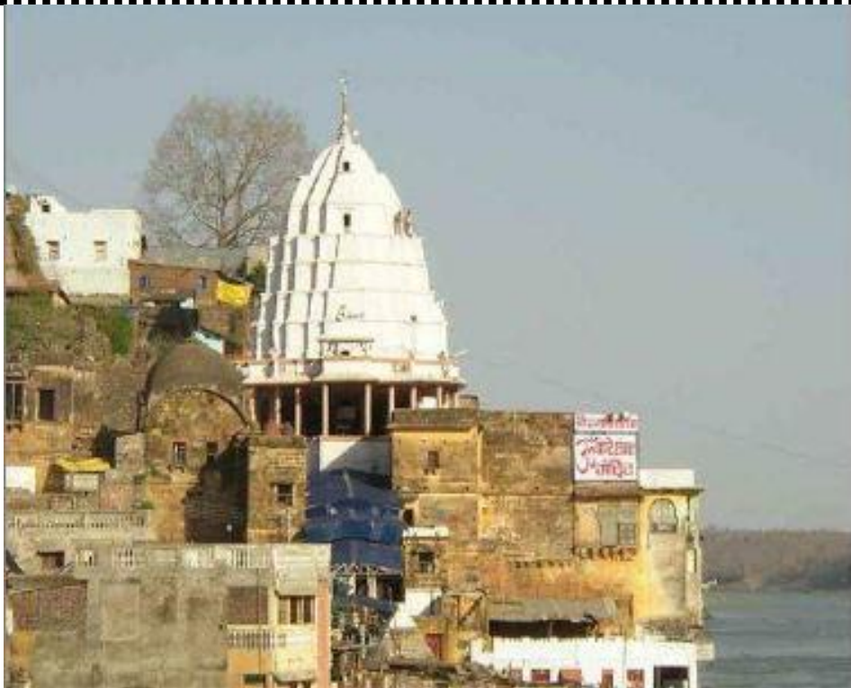
Fig. 38: Front of the Omkareshvara temple. We can distinguish the entry from the building covered by blue canvas, the mandapa located at the first stage (red columns) and the large white shikara. The temple is surrounded by many dwellings, belonging to Brahman families, built on the abrupt slope of the island.
