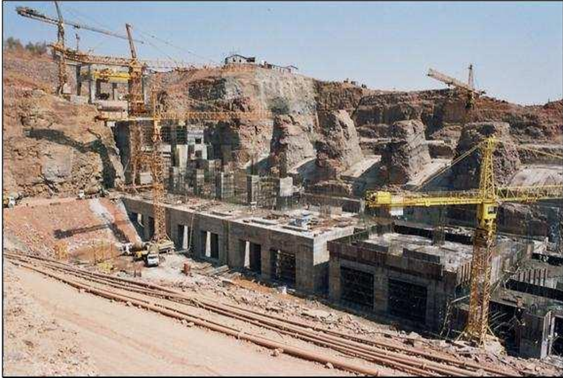
Fig. 25: Progress report of the power station (northern bank) on March 20, 2005. The SIEMENS Francis turbines will be placed in these concrete structures. Source: CREMIN Emilie, March 2005.
