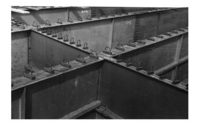
Figure 1: Steel beams with welded bar connectors for the new Herdecke Bridge (1951) over the River Ruhr (source: German Federal Ministry of Transport & Digital Infrastructure)
