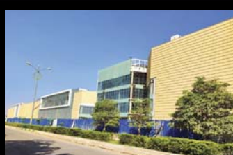
Lulu Mall, Lucknow
