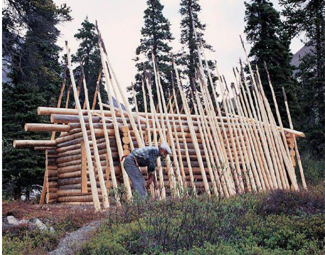
▲ ▲ Dick readies the roof poles for installation.
