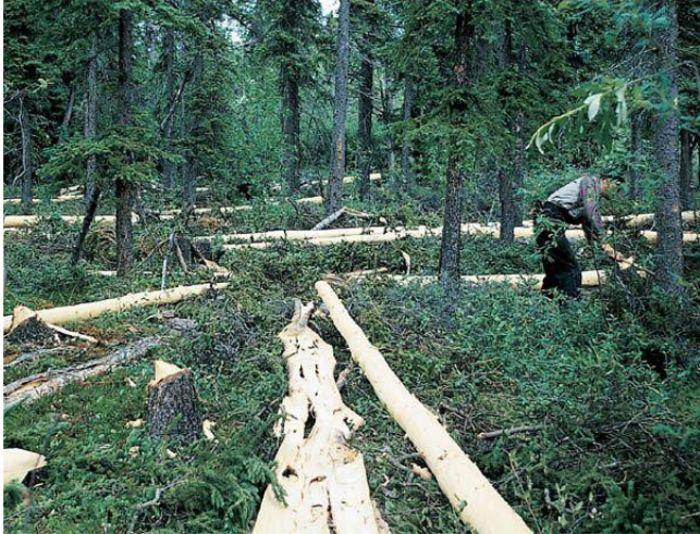
▲▲ Felling and peeling the white spruce cabin logs.
