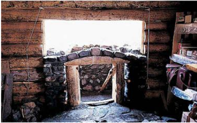
►My fireplace form is in place to support the arch.
