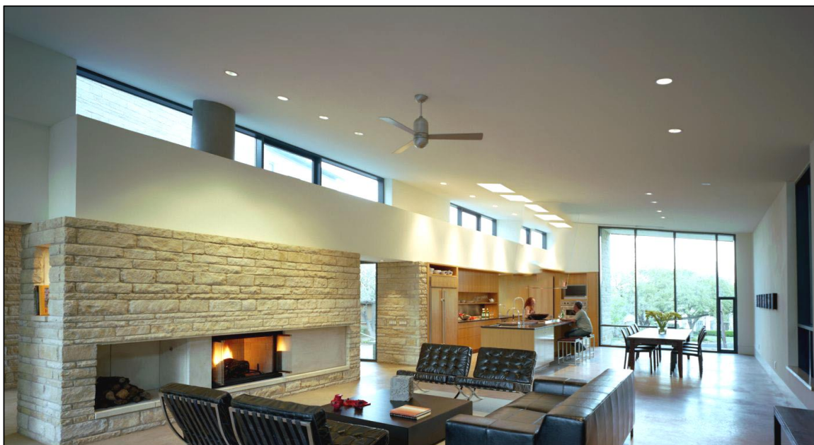
Fig. 2.3: No beam, free layout and large windows create bright and open spaces in flat slab floors
