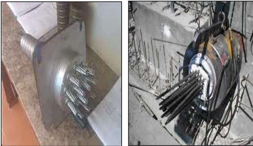
Fig. 7.3: Prestressing strands and bar
