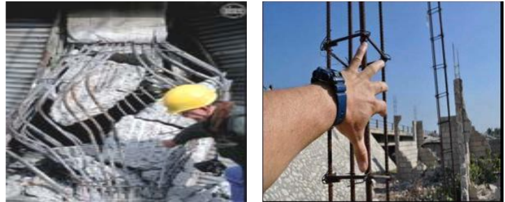
Fig. 3.3: Columns without adequate ties in earthquake
