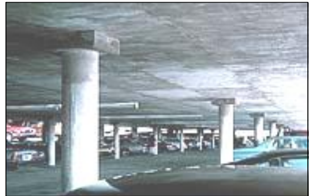
Fig. 2.2: (a) Flat plate in an office building, (b) Flat slab in a parking structure
