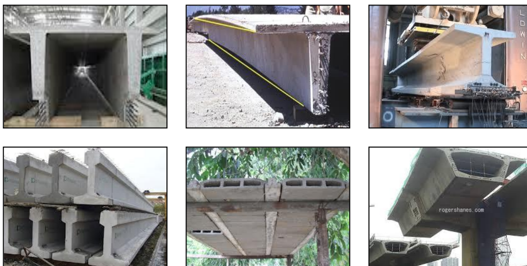
Fig. 7.5: Typical PC Sections
