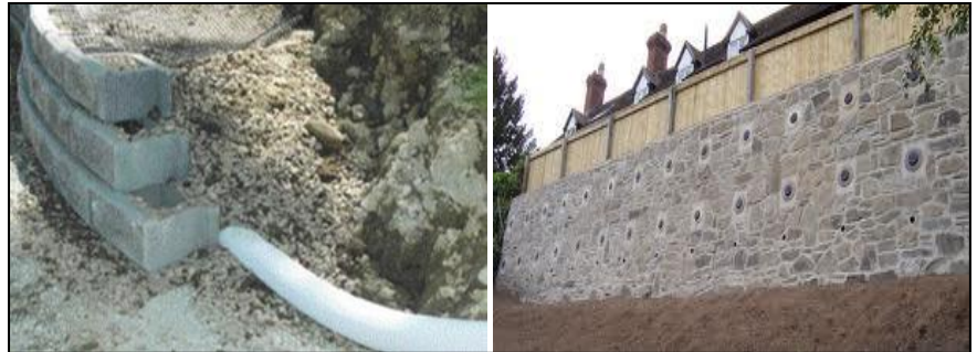
Fig. 6.4: (a) Granular soil and Tube, (b) Weep holes in retaining wall
