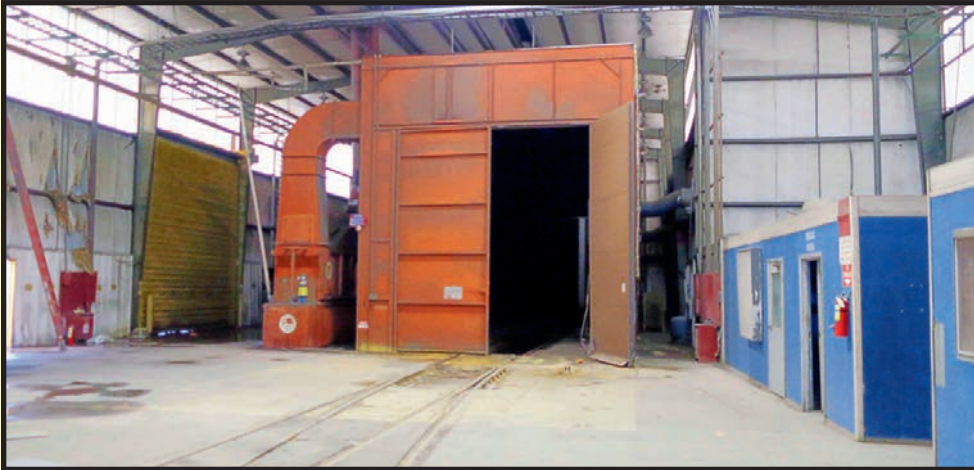
CAB SYSTEMS RAILCAR BLAST FACILITY
