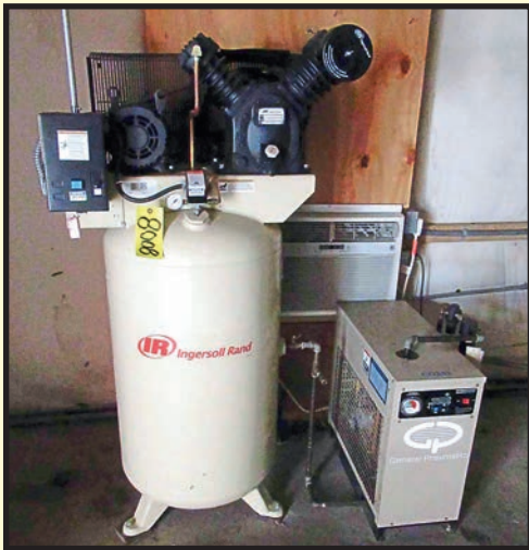
INGERSOLL RAND RECIPROCATING AIR COMPRESSOR AND DRYER SYSTEM
