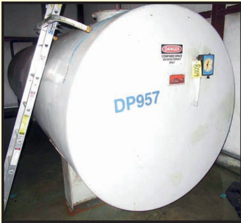
MODERN WELDING CO. INC. WATER TANK
