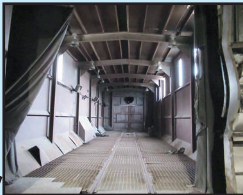
24' X 75' BLAST ROOM
