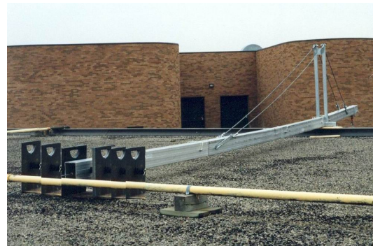
Cable Truss System
