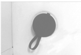
Fig. 13: Plastic plug for condensation drain (the plug seals the tank from the inside)
