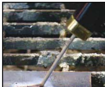
(7) To finish the weld, break the arc by quickly snapping the electrode away from the work piece.
