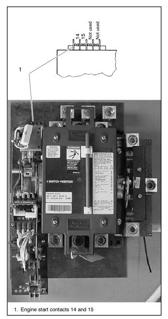
Figure 2-22 Engine Start Contacts, 225–400 Amp Open-Transition Models
