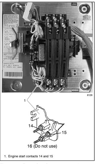
Figure 2-21 Engine Start Contacts, 30–200 Amp Switches
