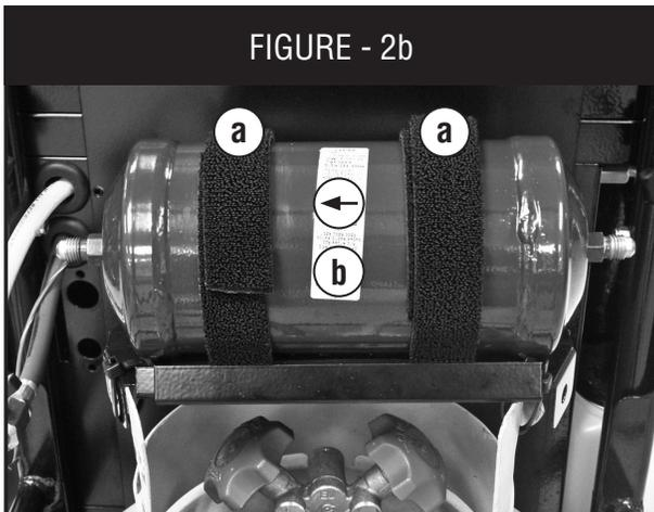
Filter placed on filter bracket
