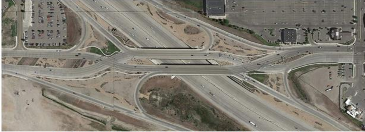
(a) Junction of Interstate 15 and State Route 92, Lehi, Utah (DDI)
