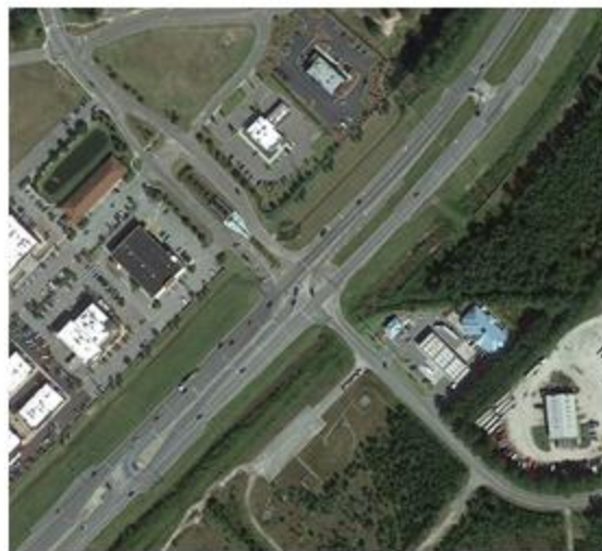
(c) Junction of Ocean Highway East and Ploof Road, Leland, North Carolina (RCUT)
