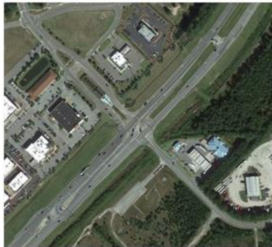
(c) Junction of Ocean Highway East and Ploof Road, Leland, North Carolina (RCUT)
