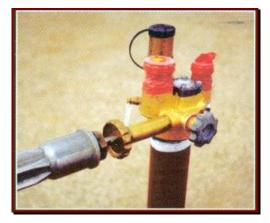
Figure 5.1.9c - Pressurizing New Vacuum Purged ASME Tank with Propane Vapor
