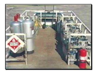
Figure 5.1.6b – Vertically Secured Cylinders
