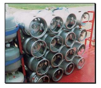
Figure 5.1.6c – Horizontally Secured Cylinders (Relief Valve at Top)
