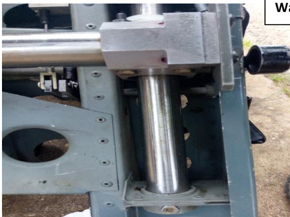
Figure 20: Missing Washer(Packers) on Captains Seat
