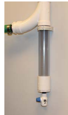
Figure 4.7-3: Drain Drip Leg
