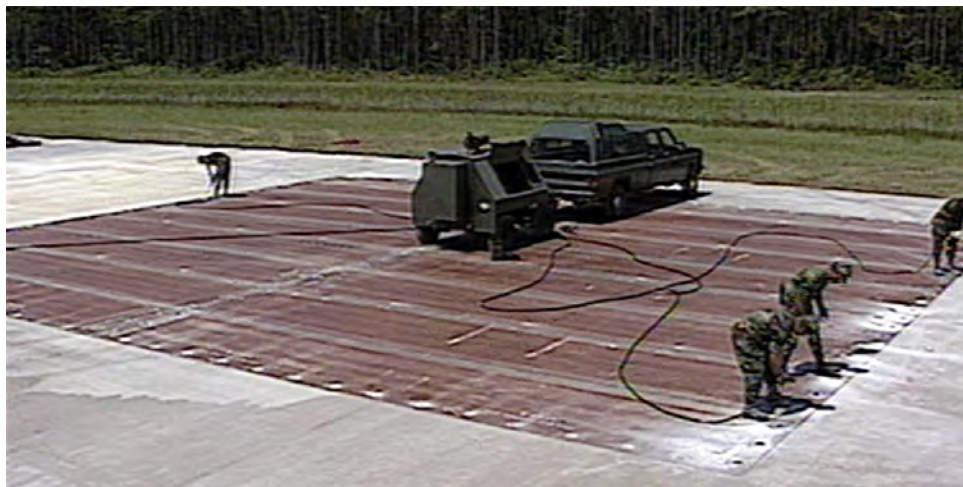
Figure 10.5. FFM Repair Method.
