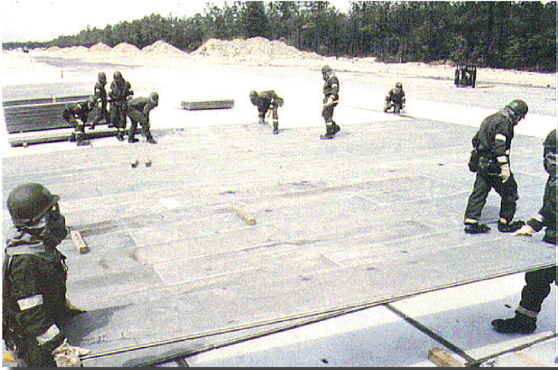
Figure 10.4. AM-2 Mat Repair Method.
