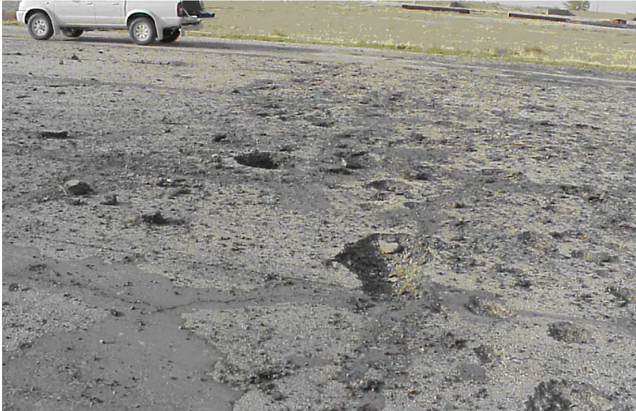
Figure 9.1. Spall Damage.
