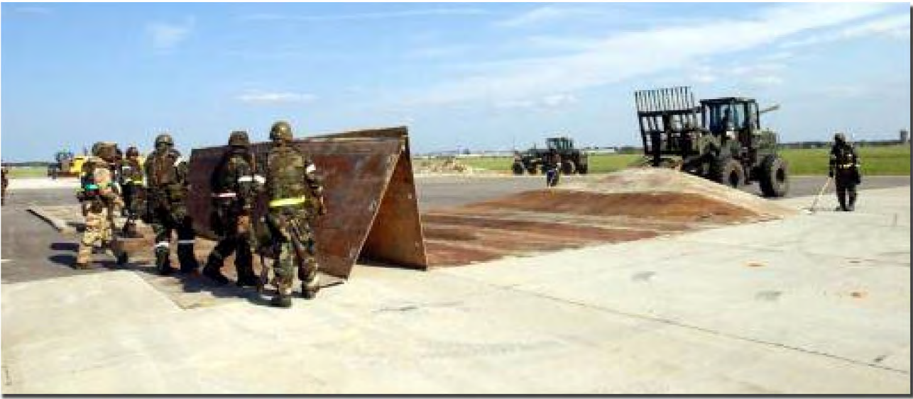
Figure 1.1. Airmen Laying Out Folding Fiberglass Matting.
