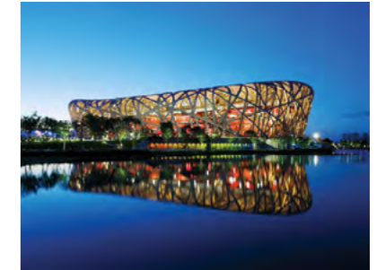
■ National Stadium (Bird's Nest)—Flame-resistance Cable
