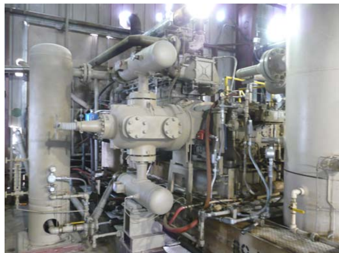
Fig. 29: Obsolete KOCA/2 frame with new Ariel cylinders applied.
