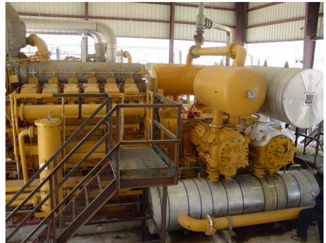
Fig. 26: 2000 hp (1491 kw), 900 rpm, gas engine driven 3-stage propane refrigeration compressor.
