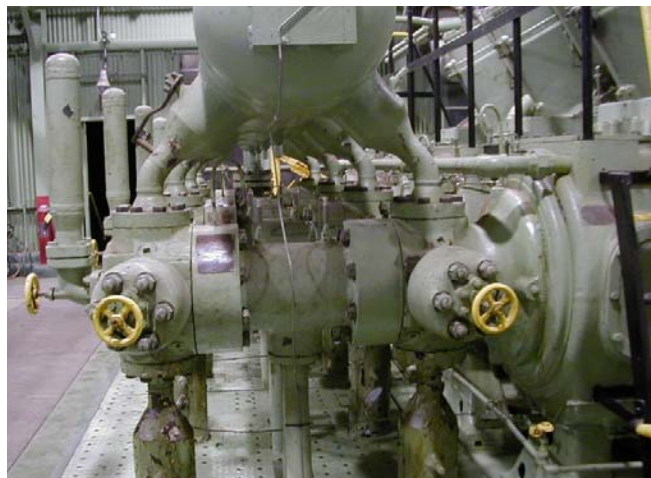
Fig. 15: Original problematic valve-in-head cylinders required disturbing the outboard piping connections to access the piston, piston rod and packing.
