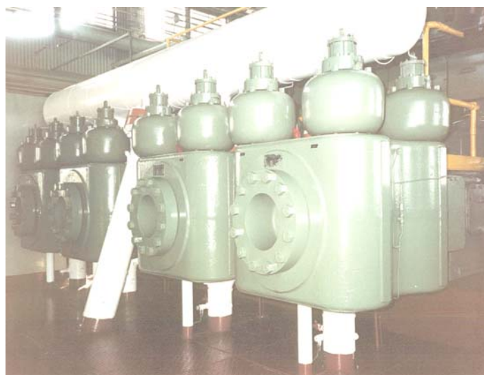
Fig. 3: Retrofitting custom engineered cylinders increased bore size by 32% on this 17 in. (431.8 mm) stroke Clark integral compressor.
