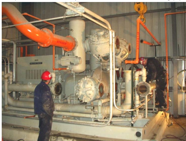
Fig. 30: Prior to reconfiguring, this oversized 3-stage Joy WB14 nitrogen compressor required 76% of the flow to be recycled.
