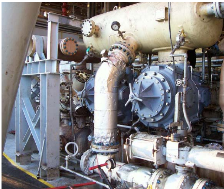
Fig. 11: New 21.0 in. (533.4 mm) bolt-in 1 st stage replacement cylinders with manual variable volume clearance pockets.
