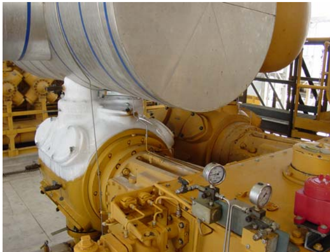
Fig. 25: Adaptation of 5.5 in. (140 mm) stroke Ariel cylinders to a Superior 6.0 in. (152 mm) stroke Superior compressor frame.
