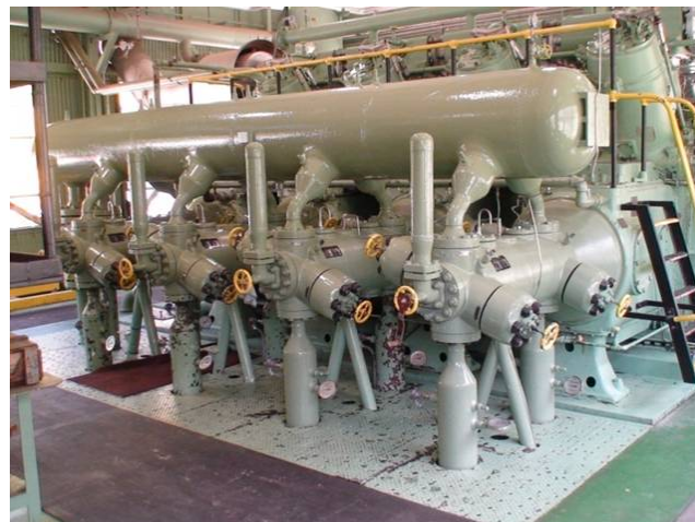
Fig. 16: New bolt-in replacement valve-in-barrel cylinders reused original valves, packing and cylinder unloaders. Piping connections are no longer disturbed for piston, rod and packing maintenance.
