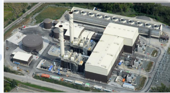
Empire Power Station GTCC, 635 MW Rensselaer, NY, US
