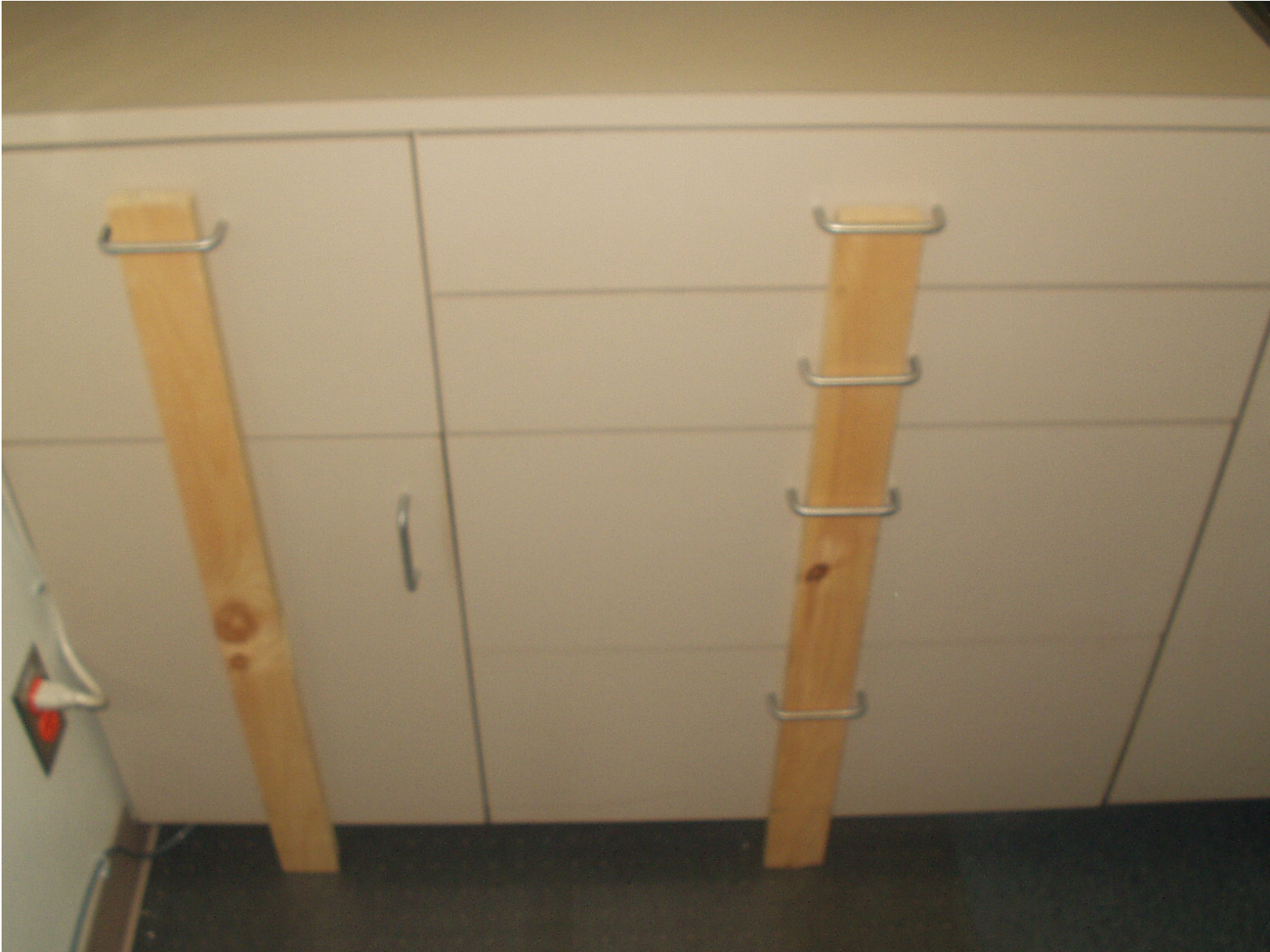
LOWER CABINETS: Secure lower cabinets and drawers for travel with the wooden bars, as shown.
