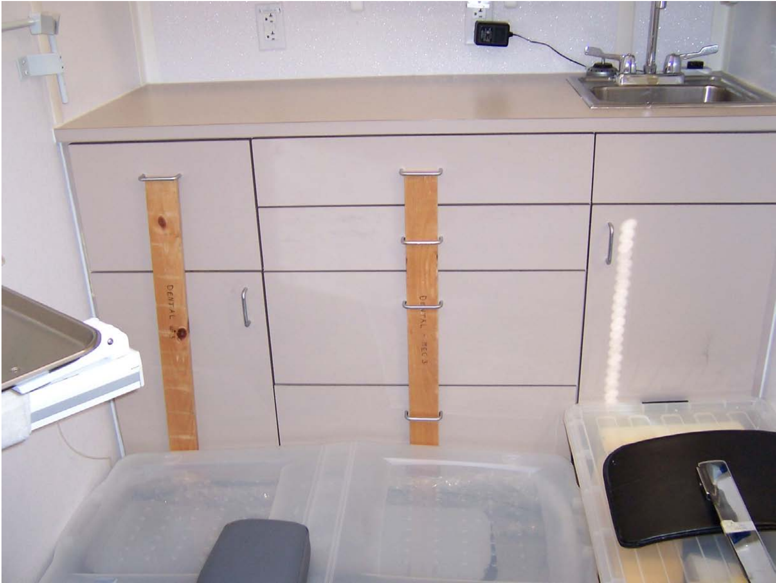
DENTAL ROOM STORAGE: Close-up showing cabinets secured with wood bars and floor storage.
