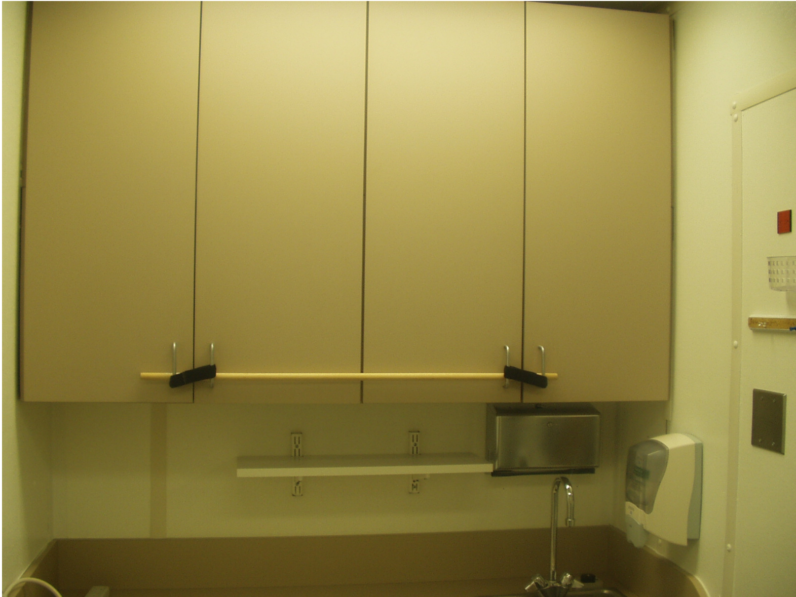
DENTAL ROOM CABINETS, SHELF AND COUNTERTOP: Remove all items from shelf above sink and countertop. Secure cabinet doors as shown with the dowel and Velcro strips.
