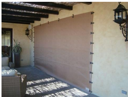
Example: large slider on a lanai with fabric in place.
