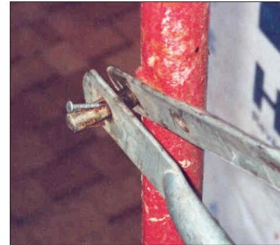
Effective inspections can detect a variety of hazards. Here, a nail is used to hold a railing in place.
