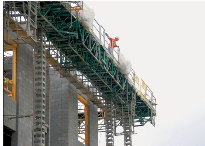
Mast climbing scaffold
