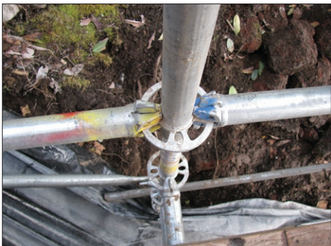
This ring rosette on a systems scaffold offers easy connections.
