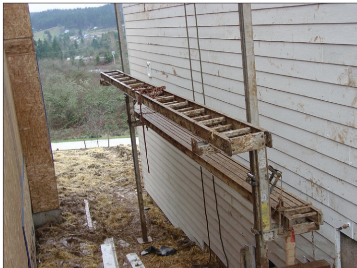
Pump jack scaffolds will normally have a work bench that can act as a top rail if it is 38 inches to 45 inches. Don't forget a midrail and guarding the ends.
