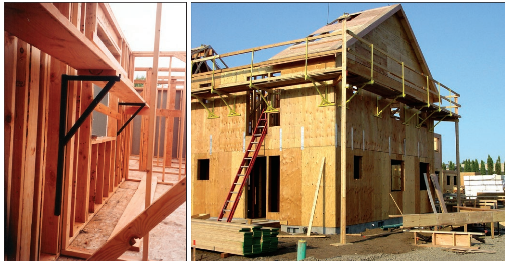
Job made (left) and manufactured carpenter's bracket scaffolding.
