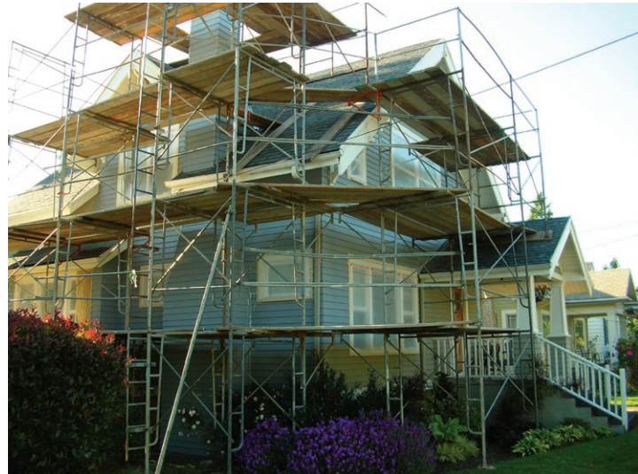
Fabricated frame scaffolds have platforms supported on fabricated end frames with integral posts, horizontal bearers, and intermediate members.
