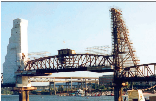
Some scaffolding jobs require much design - and planning!
