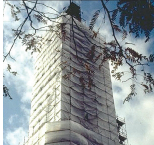
Wind screens can't be used unless the scaffold is secured against the anticipated force of the wind.
