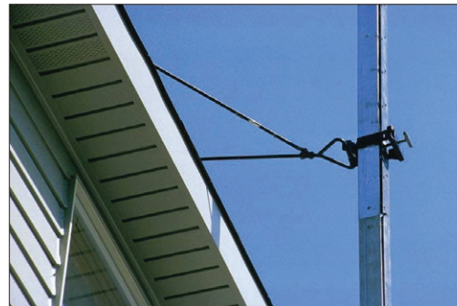
A pumpjack scaffold's triangular bracing.
