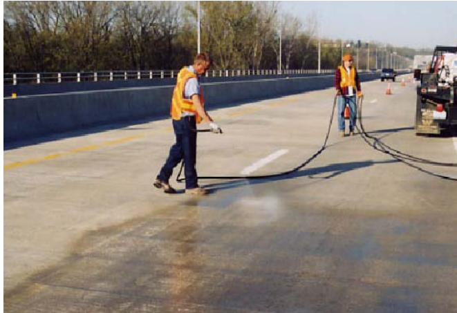
Concrete sealer being applied to test deck
