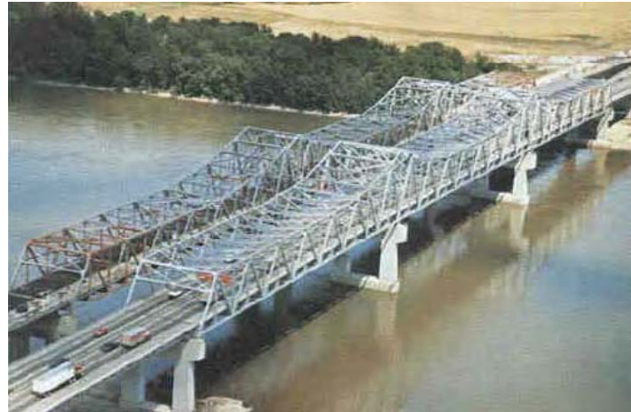
Blanchette Bridge over the Missouri River
