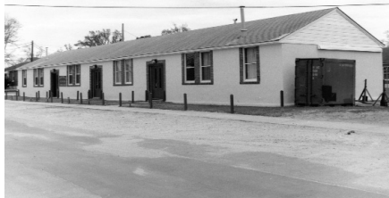
Present-day photo of one of the classroom buildings constructed at the Rifle Range. Due to wartime shortages, these buildings were constructed of stucco and clay-tiles.
