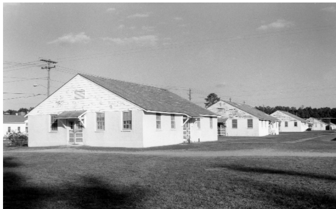
Washrooms at Montford Point Camp No. 2.
