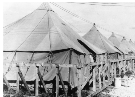
Tents on platforms at Tent Camp No. 1, 1941.
