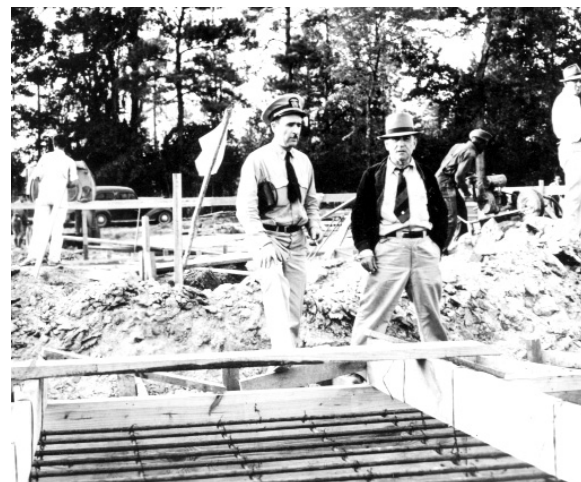
The Construction Officer inspects the progress of buildings at Marine Barracks New River.
