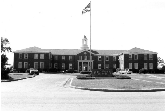
View looking southwest at Building 2, originally the Division Headquarters, now headquarters of the 2d FSSG.
