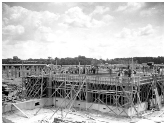
Construction of the hospital, 1941.
