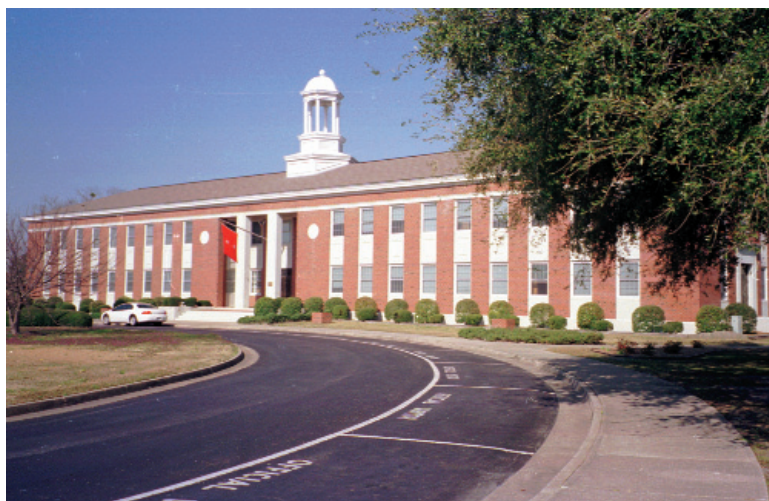
Building 1, Post Headquarters, at the corner of Holcomb Boulevard and Main Service Road.
