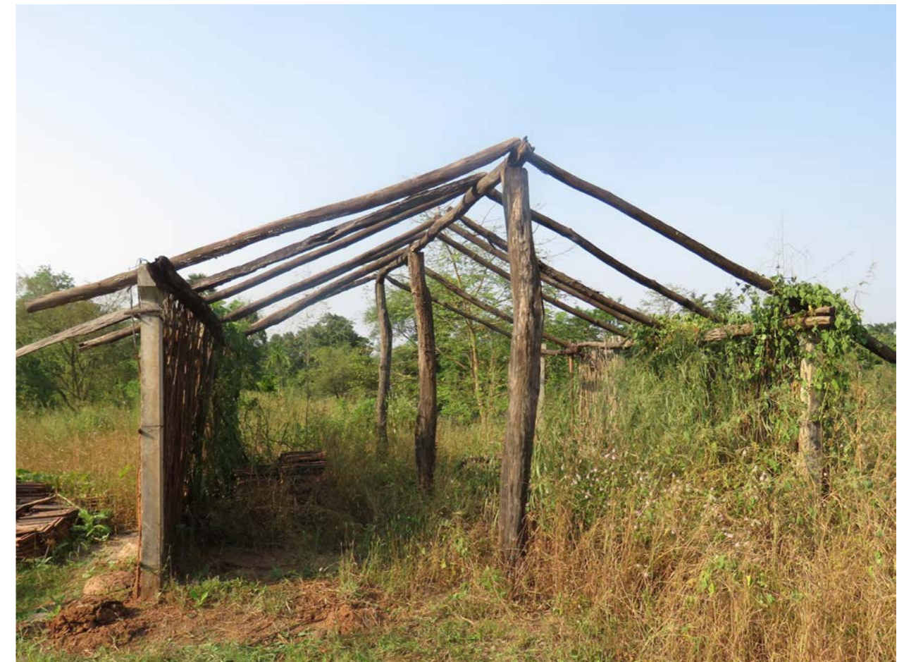
Plate 2: Warlis house framework, Dahanu, Maharashtra, India. Photograph by Rashida Atthar, 2016.
